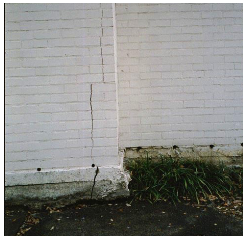
Fig. 8 Cracked foundation on home due to the shrinking and swelling of Houston Black clay it was built upon. Credit: Clay Robinson
