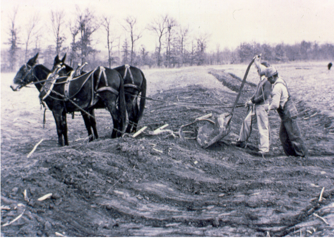
Fig. 7 Fresno Scraper was utilized to assist movement of large amounts of soil efficiently when leveling the natural microrelief of the landscape. Credit: ASME landmarks program.
